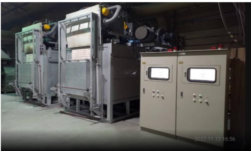
建置蓄熱式燒結爐
